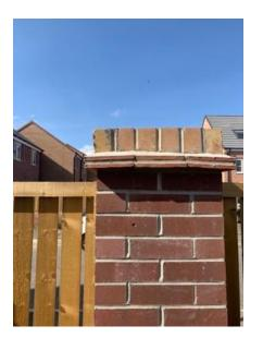
Snag 71 Location: Garden Insufficient mortar
