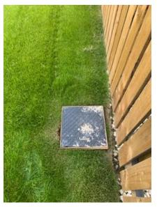
Snag 70 Location: Garden Drain cover not correctly installed
